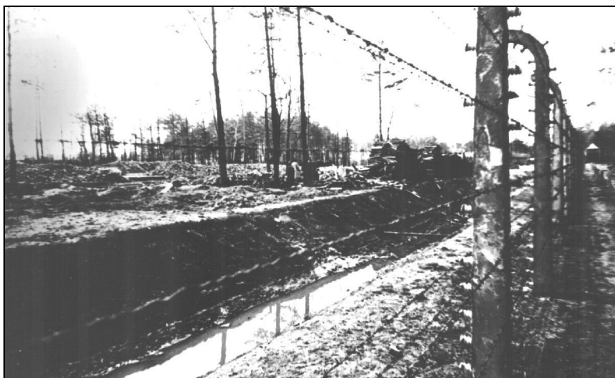
Fig. 5: Drainage ditch running north of Crematorium V.
