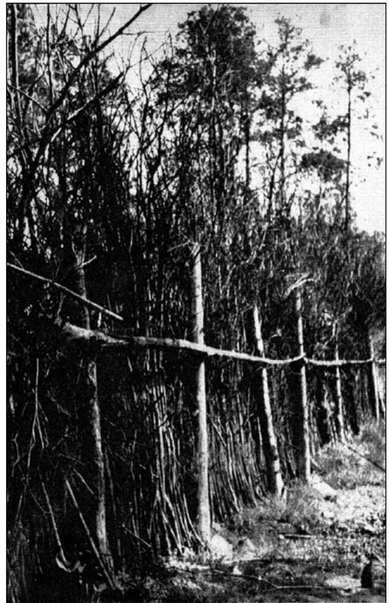
Illustration 3: “Birkenau. Part of the wicker fencing masking the crematory.”
