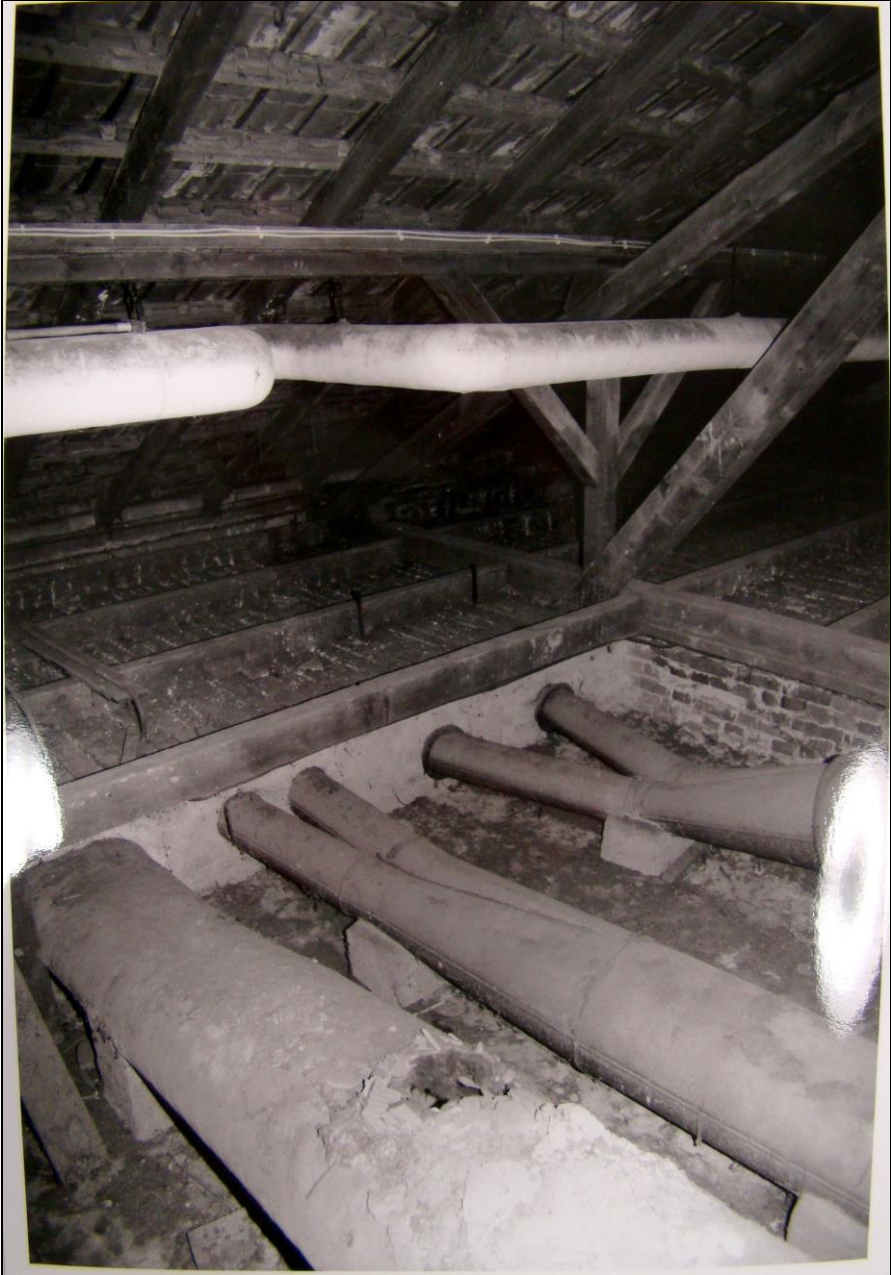
Documents 14, 14a (labeled): Photo by R. Müller showing the attic of the Dachau Crematorium above Room 8 and 9 (1995). Source: Archives of the Dachau Museum, Folder Krematorium Baracke X.
