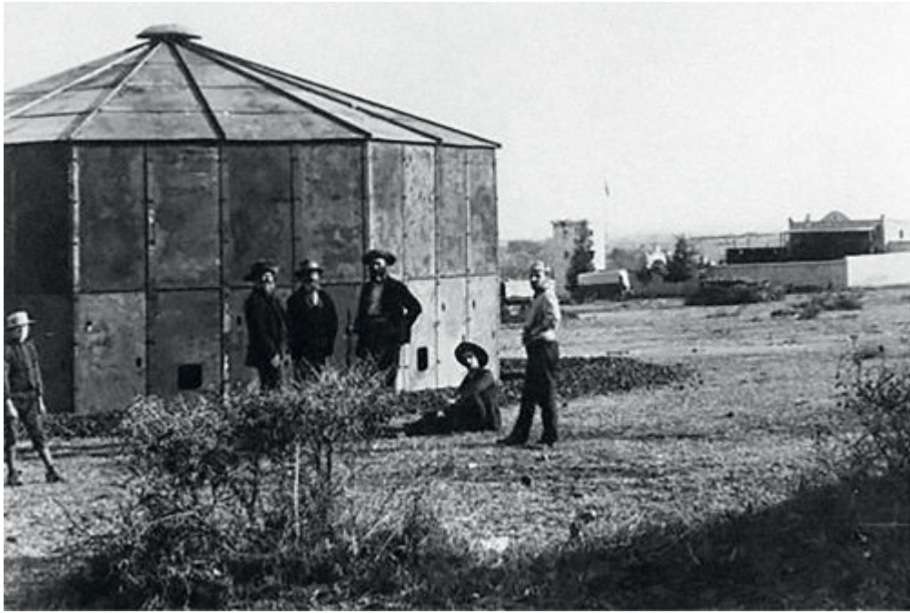
Fort Edward, the pre-fabricated collapsible steel fort used by the BVC as a base in the Northern Transvaal. This photo was taken by H.F. Gros, c. 1888, prior to the war, when the fort was known as Fort Hendrina.
