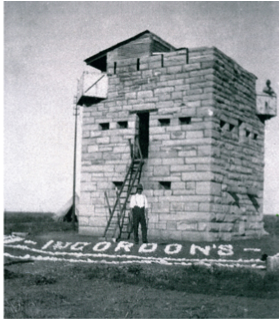
A stone blockhouse fort, one of up to 8000 constructed and garrisoned by the British to guard rail lines and other key infrastructure during the war. (Alamy)
