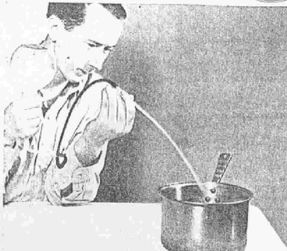
You can make an experimental fire extinguisher that works on the same principle as the commercial type. It squirts a stream of water as below
