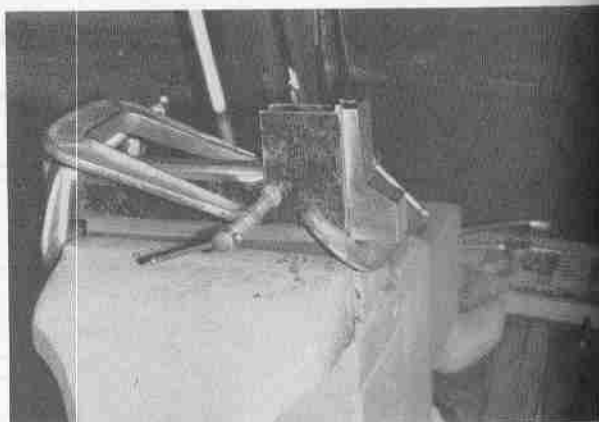
Clamped in place for welding. Note that a filler block is inserted to keep the assembly square and maintain dimensions.
