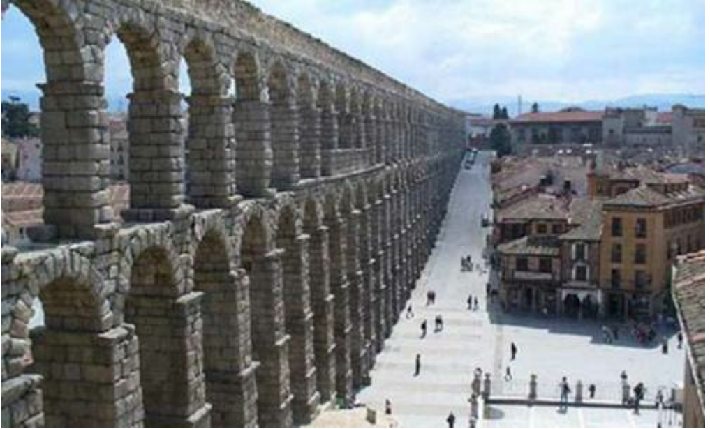
A tribute to Roman engineering—the Roman-built aqueduct at Segovia in Spain.
