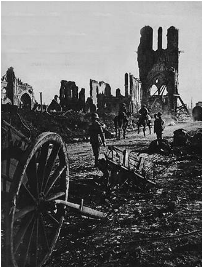
The staggering scale of the destruction wrought on the western front, caused by continuous bombardment of the same positions due to the largely static front line, is evident from this photograph of the remains of a French town, situated just behind the Allied front. Some areas were leveled to the ground: trees, grass, shrubs, and buildings alike.
