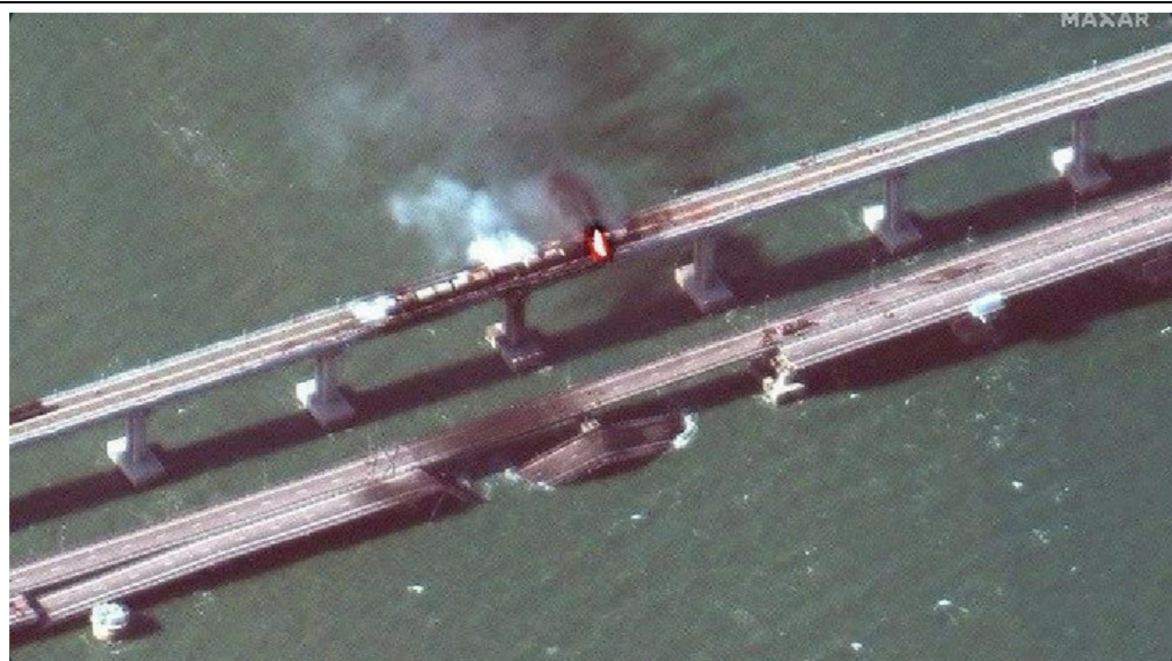
Aerial view of the damage to the Crimean Bridge; ground zero of the explosion, burning fuel train and the damage to the three spans are visible.
