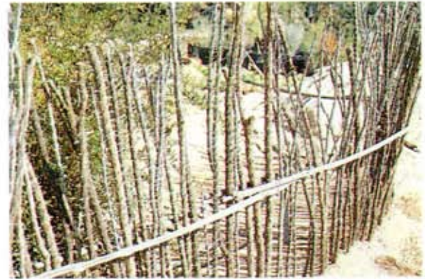
89. TUCSON, AZ, USA. A spiny Ocotillo hedge guards an O'o'dam (Papago) garden. This species is cultivated for fencing, can be liveset to grow if irrigated, and is widely used as a reinforcement or base for mud wall construction. It is a useful crop in itself for desert structures.
