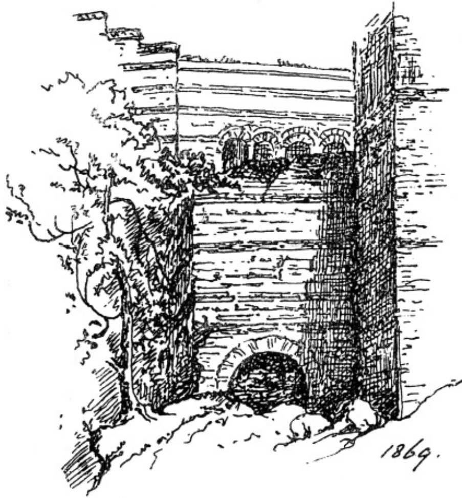
The blocked-up arch of the Circus Gate
