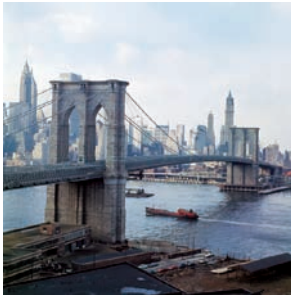
27-46A ROEBLING, Brooklyn Bridge, 1867–1883.
