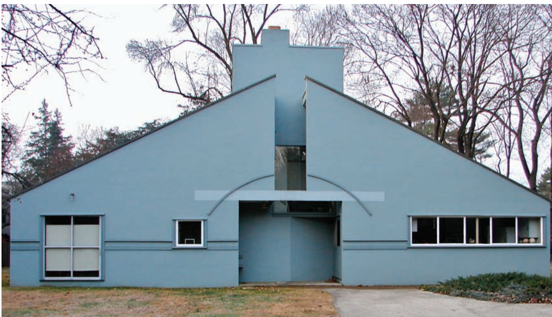
30-48 Robert Venturi, Vanna Venturi House, Chestnut Hill, Pennsylvania, 1962.
