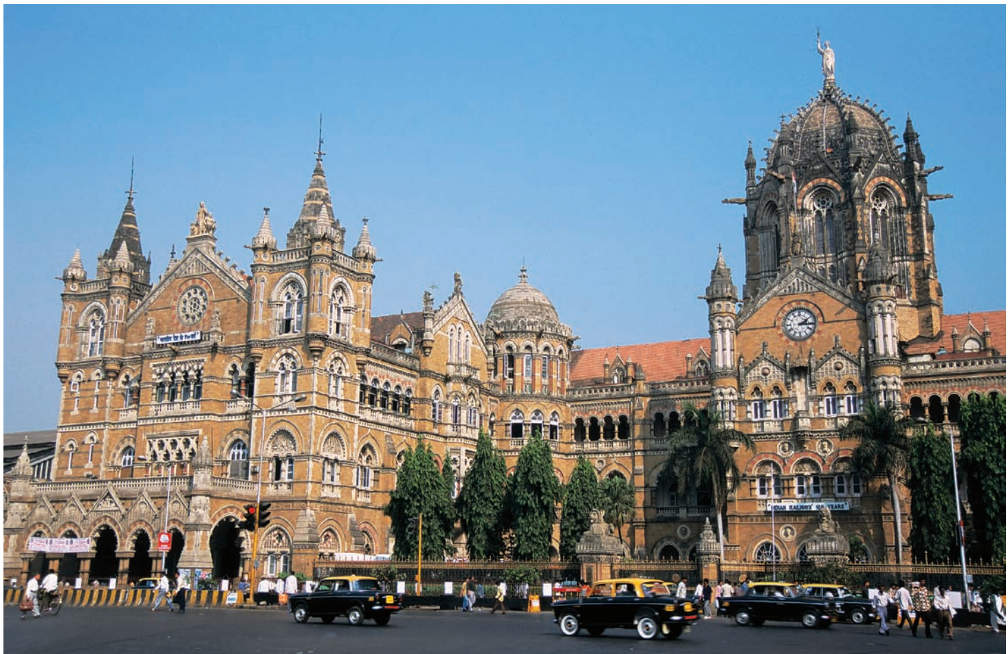
32-9 Frederick W. Stevens, Victoria Terminus (now Chhatrapati Shivaji Terminus; looking northeast), Mumbai (Bombay), India, 1878–1887.
