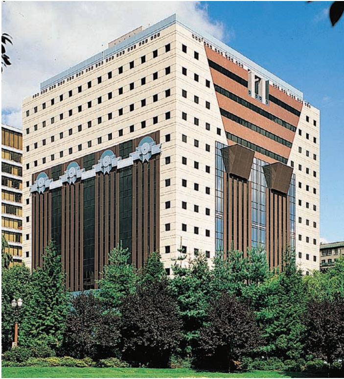
30-47 Michael Graves, Portland Building (looking northwest), Portland, 1980.
