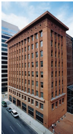
28-40A SULLIVAN, Wainwright Building, St. Louis, 1890–1891.
