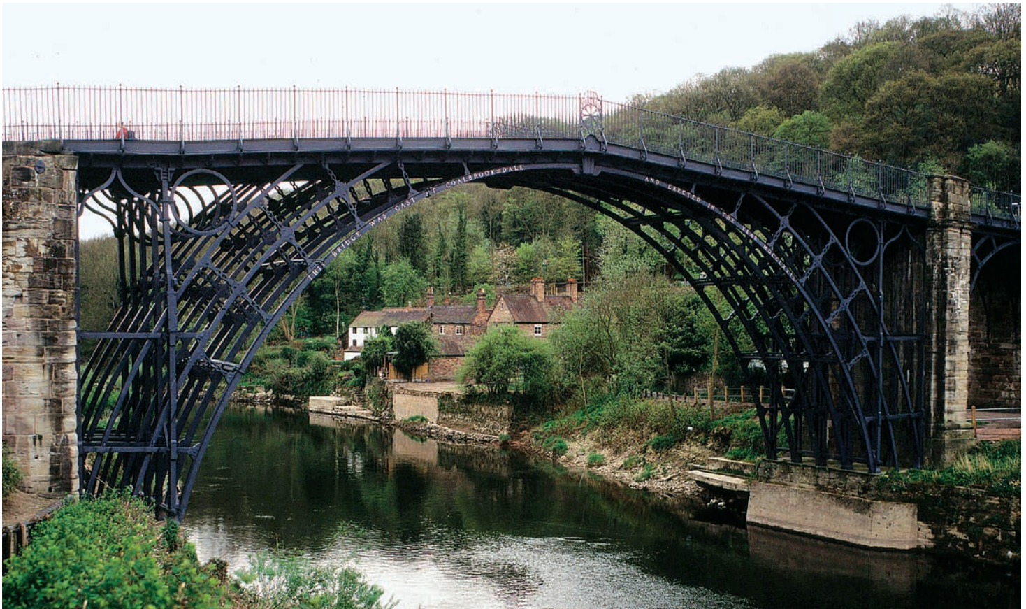
26-12 Abraham Darby III and Thomas F. Pritchard, iron bridge (looking northwest), Coalbrookdale, England, 1776–1779.
