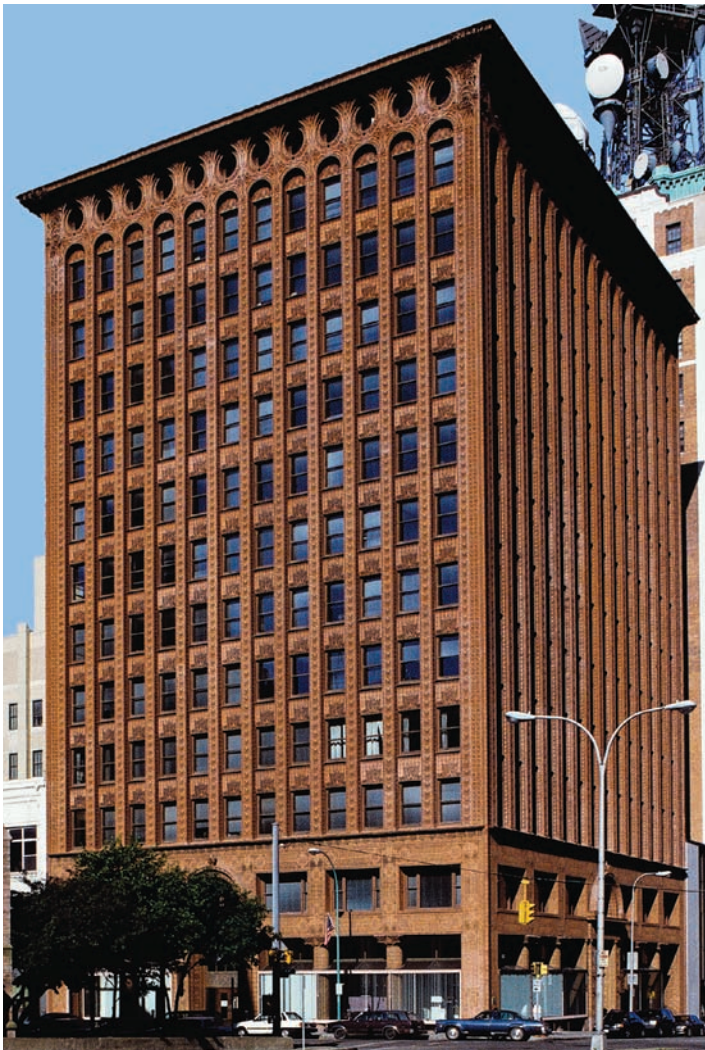
28-40 Louis Henry Sullivan, Guaranty (Prudential) Building (looking southwest), Buffalo, New York, 1894–1896.
