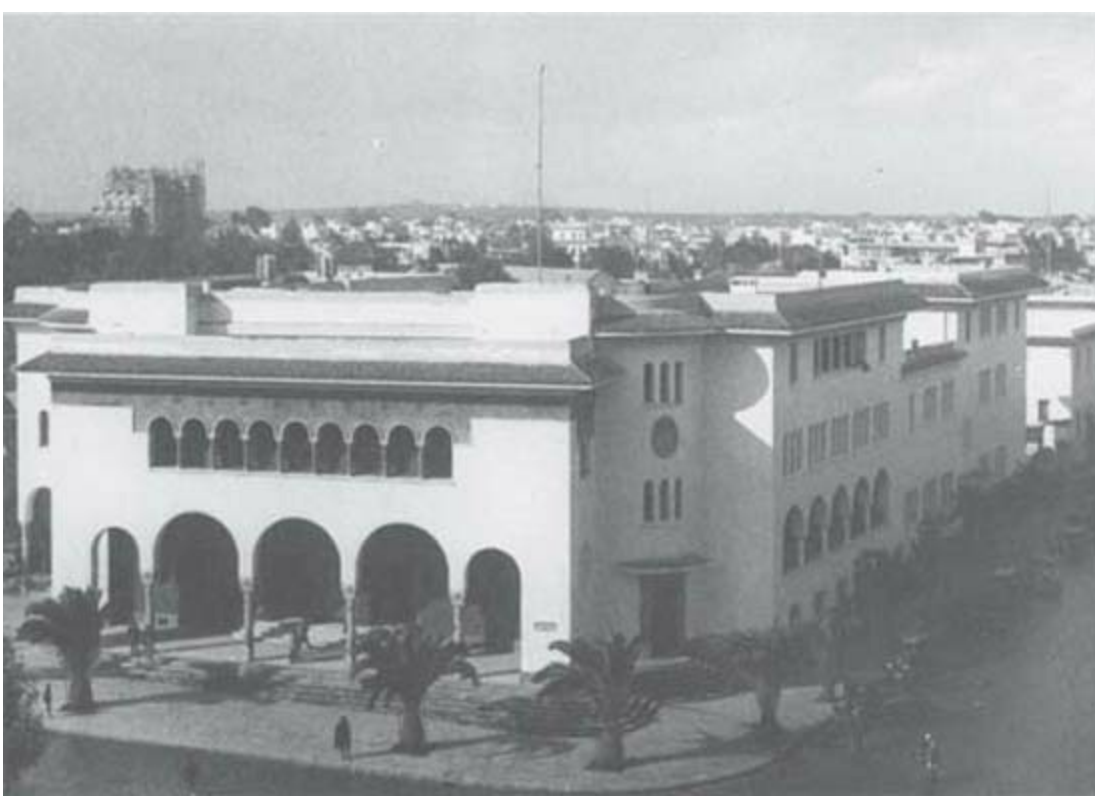
PLATE 40.1 Central Post Office, Casablanca, by Adrien Laforgue, 1920. (From Henri Descamps, L'Architecture moderne au Maroc , 1930. Reproduced in Gwendolyn Wright, The Politics of Design in Colonial Urbanism (University of Chicago Press: Chicago, 1991), 109.)
