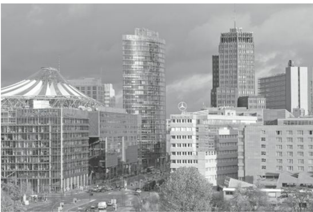
PLATE 25.2 Potsdamer Platz. After the removal of the Berlin Wall in the early 1990s, the area became one of the world's biggest and most creative construction sites. Dozens of new buildings were erected in a part of the city that, for many years, had been a desolate no-man's-land. (Source: Bildarchiv Preussischer Kulturbesitz.)
