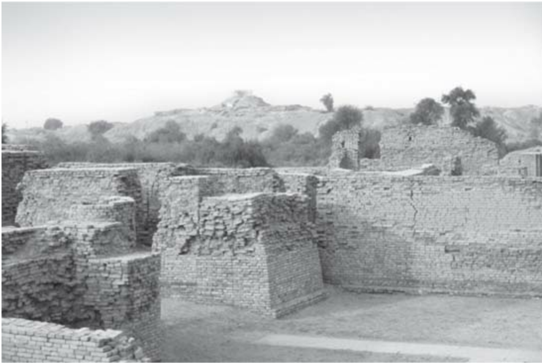
PLATE 5.1 Fired brick architecture at Mohenjo-daro, showing House VIII in HR-A area with the so-called Buddhist stupa in the background. This structure stands on the highest point on the site and dominates the Mound of Great Bath.
