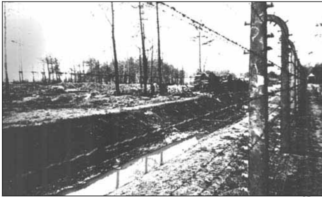
Fig. 5: Drainage ditch running north of Crematorium V 25
