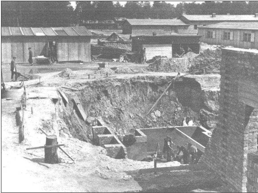
Fig. 3: Excavation work for the foundation of the Central Sauna in May 1943.
