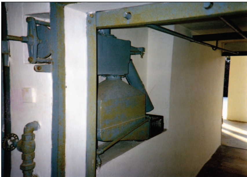
Document 13: Photograph of metallic recirculation device of a disinfestation chamber using HCN gas (Zyklon B) with the Degesch-Kreislauf system at the Dachau camp. © Carlo Mattogno 1990.
