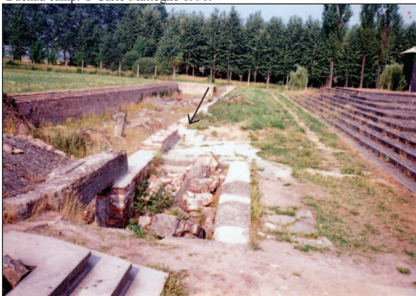
Document 14: Photograph of the ruins of Crematorium II at Birkenau, 1992. © Carlo Mattogno.
