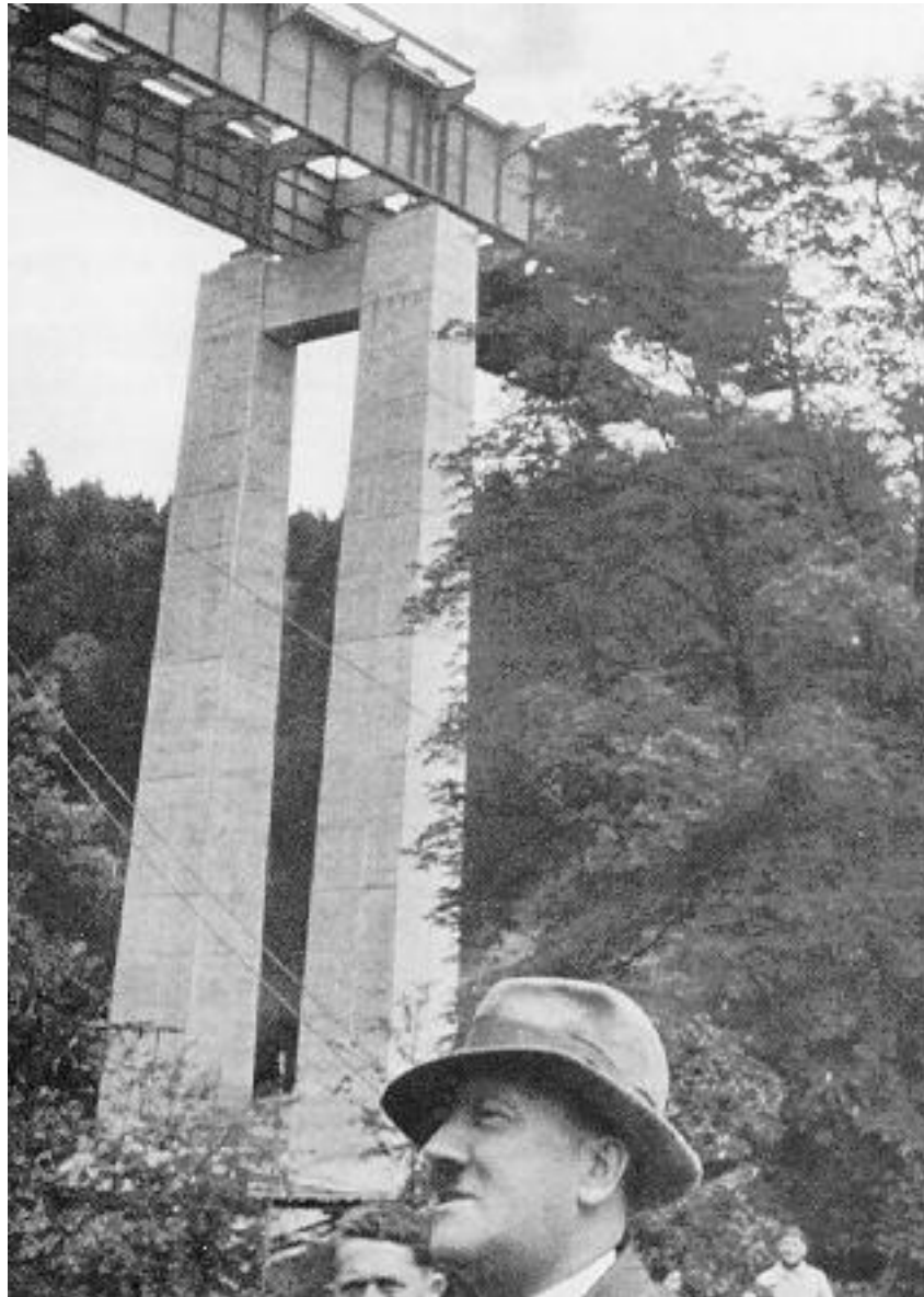
In summer, 1935, at the Mangfall Bridge.
