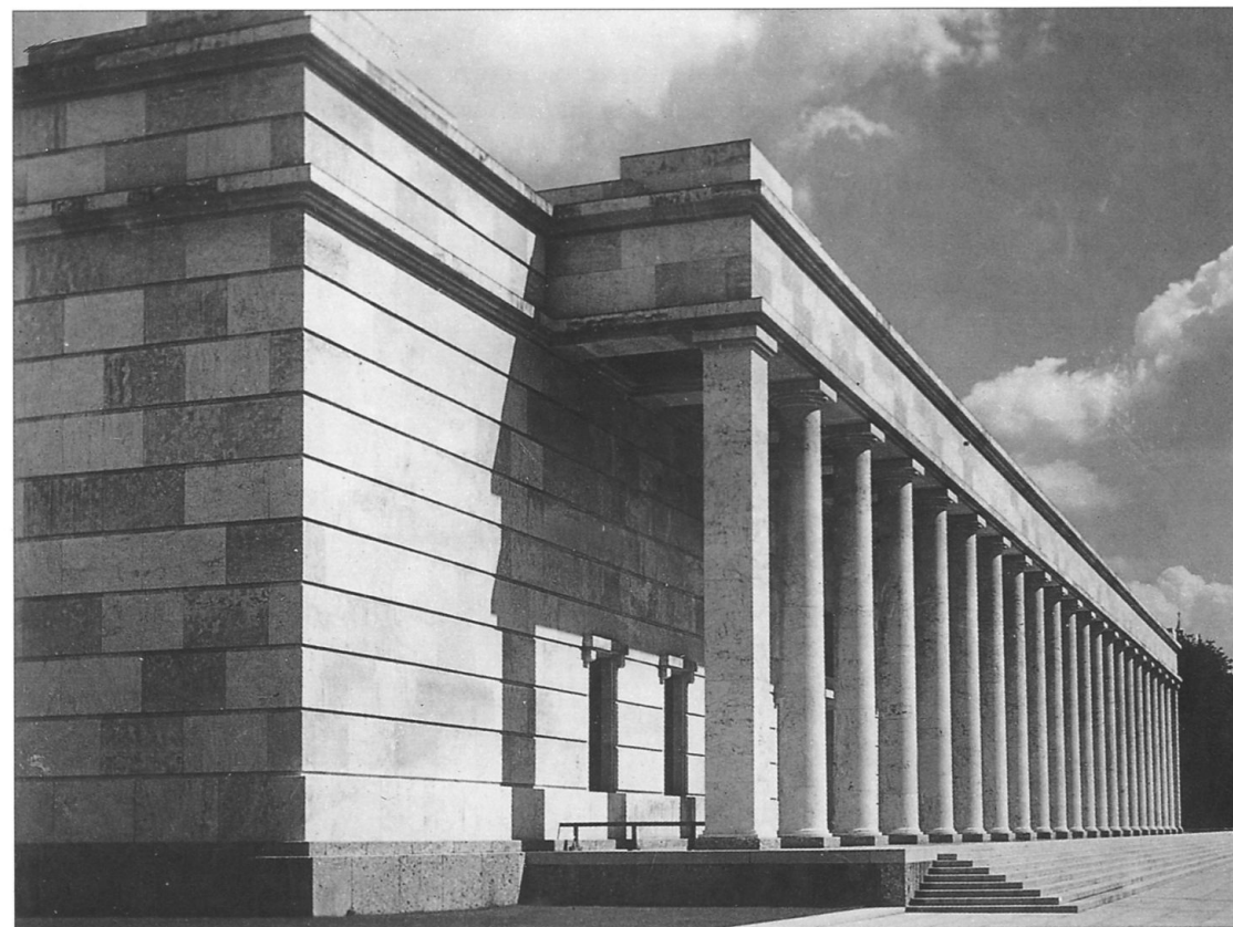
Below: The Haus der Deutschen Kunst (House of German Art) was one of Hitler's first building projects. The museum was designed by Paul Ludwig Troost, who did not live to see its opening in 1937.
