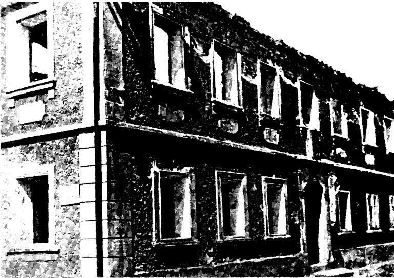
Derelict German School in Eger-Karlsbad District.
