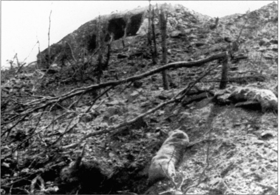
One of the bunkers of the Metaxas Line, destroyed by Gebirgsjäger during the campaign in Greece, 1941.
