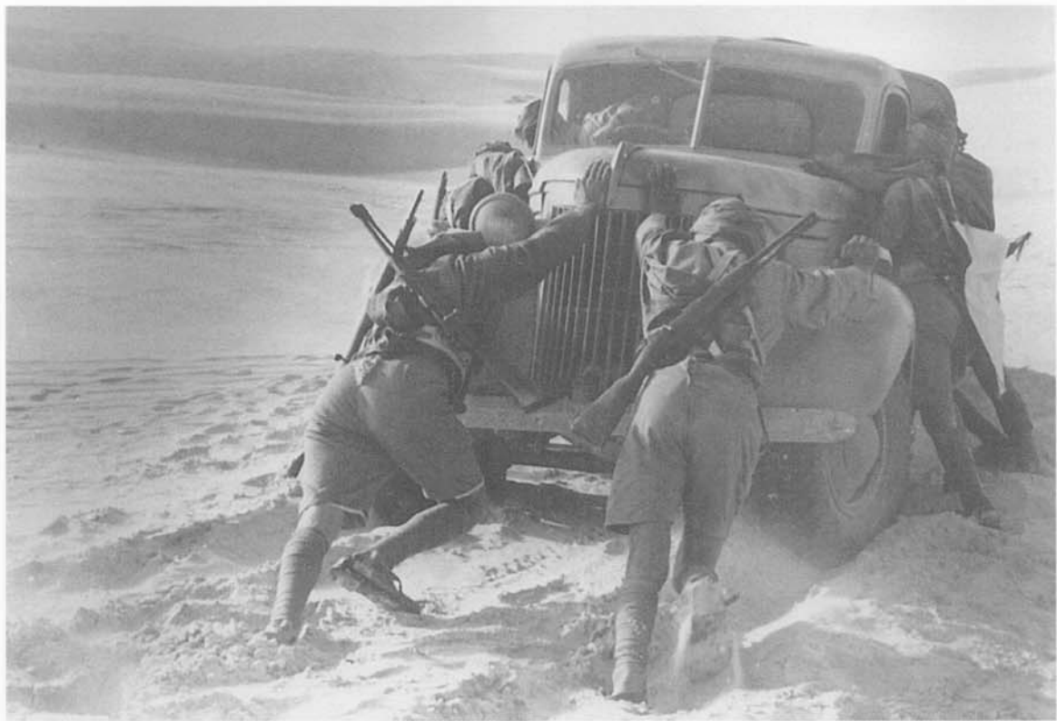
The desert sands were a continual problem to both sides. Here some Italian soldiers struggle with a small lorry stuck in soft sand. They do not appear to be using sand channels, which were essential equipment for every wheeled vehicle. (Officio Storico, Rome, via Philip Jowett)
