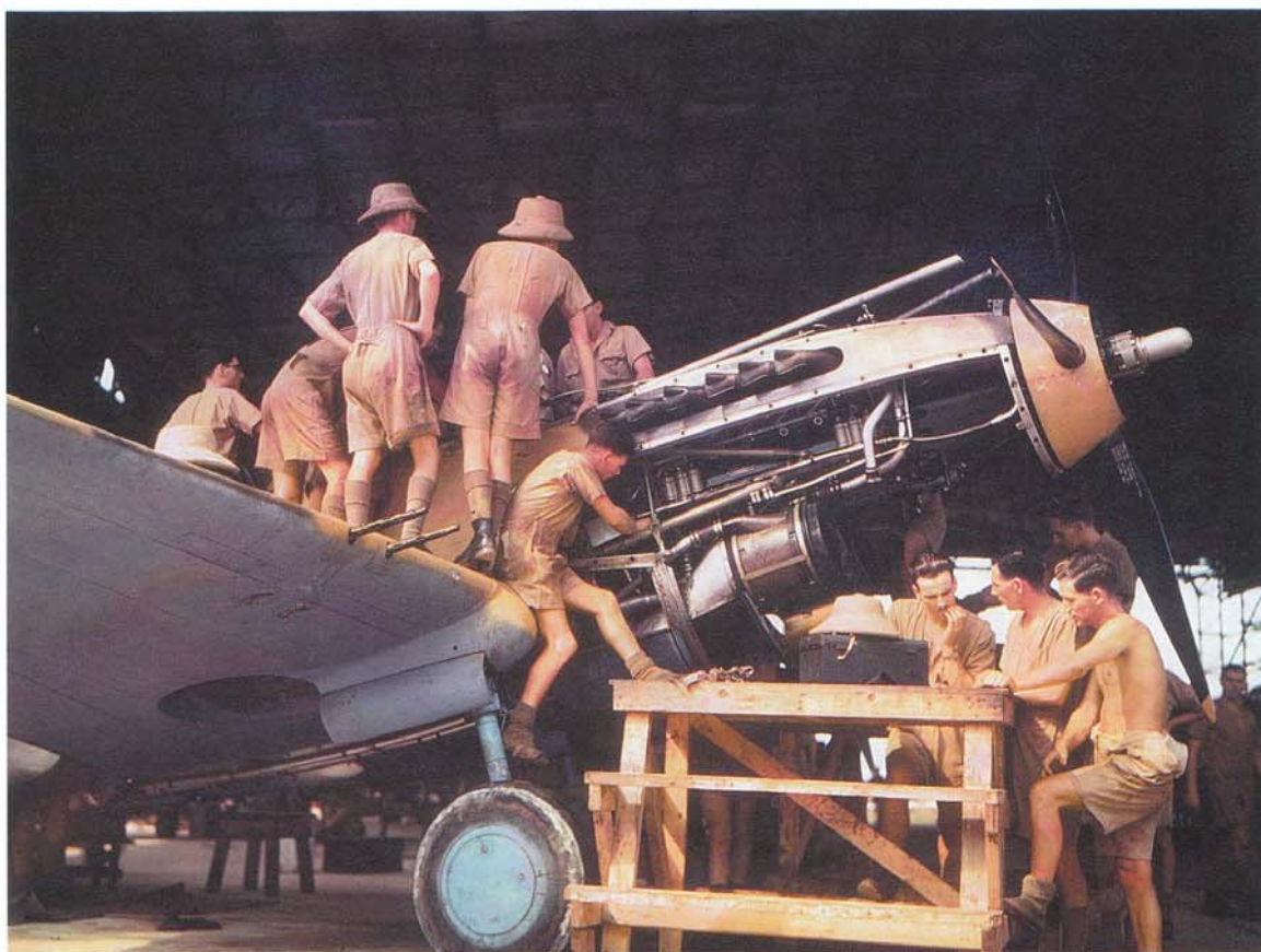
Ground crews working on the Allison engine of a Tomahawk fighter aircraft of the Desert Air Force inside a makeshift hangar. (IWM – TR 824)
