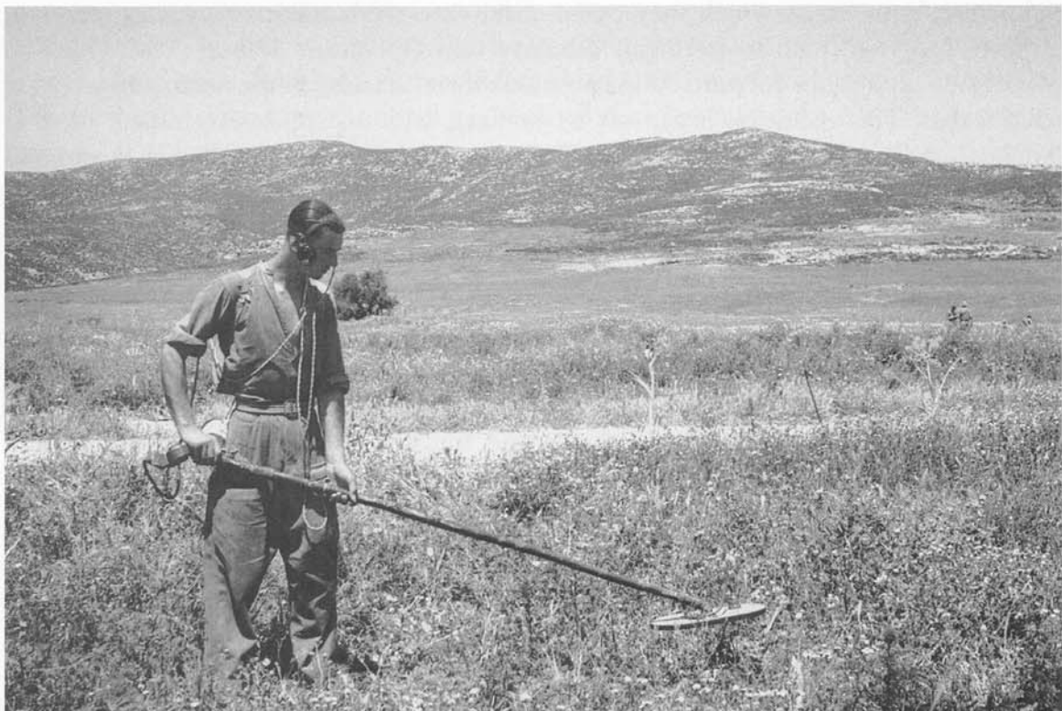
Sweeping for mines at the side of the Medjez—Tebourba road, April 1943. In the background is Longstop Hill. Some four hundred German anti-tank mines were lifted on this road in three hours. (IWM — NA 2411)
