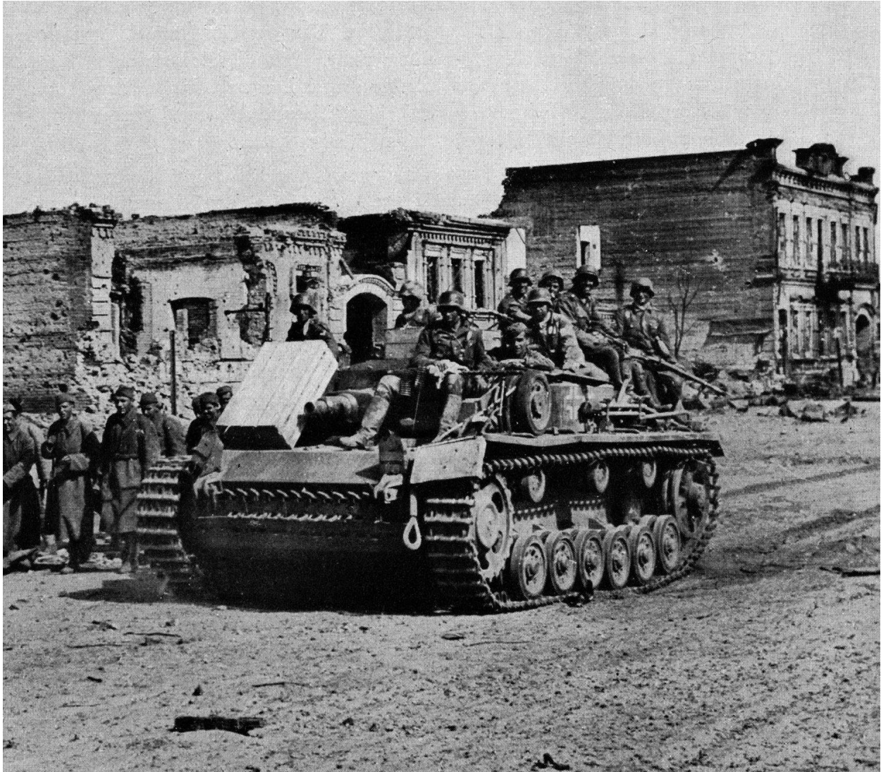
A self-propelled Sturmgeschütz III assault gun, consisting of a 75mm cannon mounted on the chassis of a Panzer III, passes Soviet prisoners in Stalingrad during the prolonged siege in late summer 1942. (Bundesarchiv)
