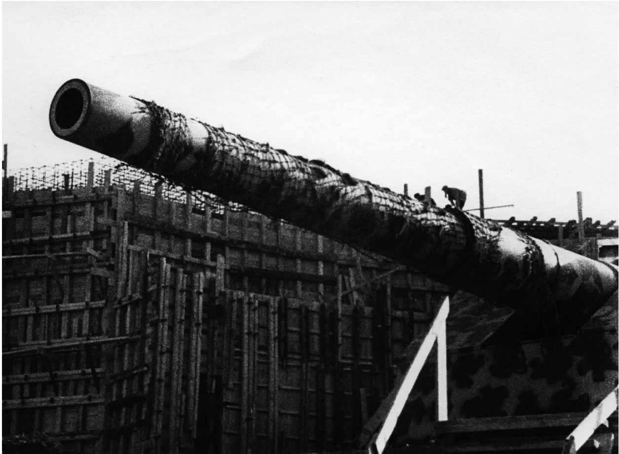
Battery Lindemann along the Atlantic Wall. The Germans constructed massive concrete shelters to protect coastal artillery from damage by Allied aerial and naval bombardment.
