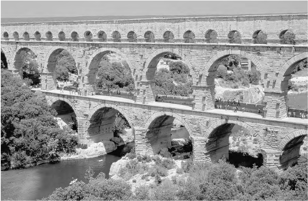
Figure 11.9 The Pont du Gard. This span, 330 feet (49 m) in height, is part of a larger aqueduct system that Agrippa sponsored to carry water to Colonia Augusta Nemausus (modern Nîmes, France) from a source 31 miles (50 km) away. In fact most of this aqueduct, like others, was underground, which was a safer and more economical method of construction. But because gravity was responsible for water flow, and siphons were generally unreliable and expensive, the water channel of an aqueduct would be carried directly across gorges, often at a considerable height, as here. This aqueduct is estimated to have had a flow of some 30,000 cubic meters a day, and to have cost up to 100 million sesterces.
